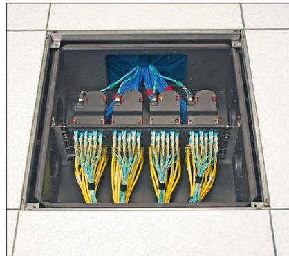
PZRFE8U with QuickNet™ Copper and Fiber Connectivity
