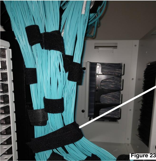
Fasten all fiber cable bundles together with one hook-n-loop
