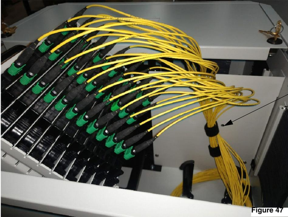
Fasten Hook-n-Loop through mounting hole in side of partition wall to cable at rear of cassette
