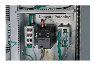
the risk of downtime associated with power interruptions to keep key equipment in facilities operating at full capacity. It is designed for critical networking and control applications such as industrial managed switches and human machine interfaces (HMIs).
