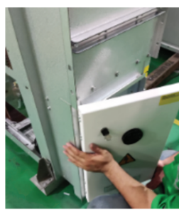
Rear cable access door secured cable access arrangement
