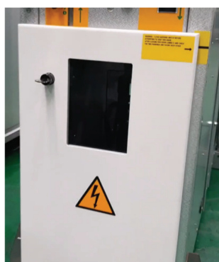
Earthing switch close key can be used for opening the rear cable access door
