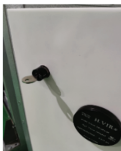
Earthing switch close key can be used for opening the rear cable access door
