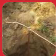
1. Copper bonded steel conductor, CBSC
