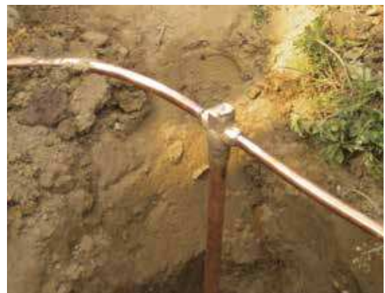
GT Cadweld connection
