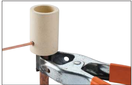
Fig. 7 – Insert the conductors and position them for the connection. To support the One Shot on the rod, use locking pliers or clamp B399P (sold separately).
