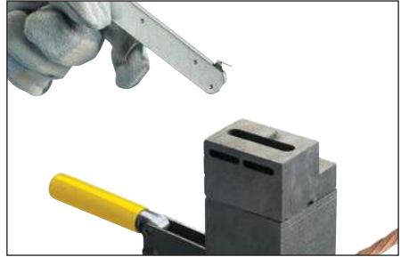
Fig. 24 – Aiming the flint igniter from the side, ignite the starting material on the mold cover. Withdraw the igniter quickly to prevent fouling.
