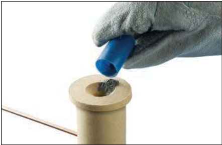
Fig. 14 – Pour the starting material onto the Cadweld One Shot cover.
