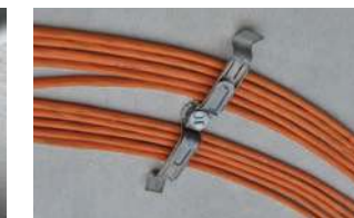
Cables from concrete ceiling / wall
