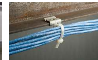
Cables from beam
