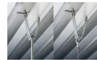
Threaded rod/chain/wire from trapezoidal steel decking
