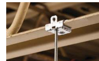
Threaded rod/chain/wire from beam
