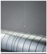
STEP 3: Attach wire rope to load.
