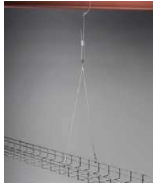
Figure 7: Speed Link Y-Hook with Eyelet Extension supporting a wire basket tray
