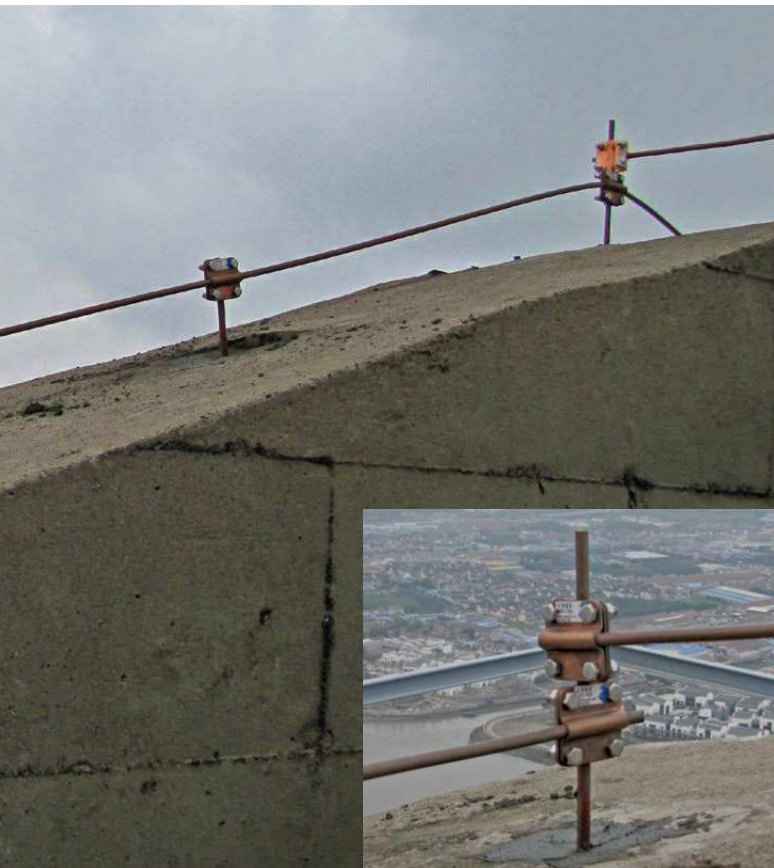
Lightning protection
