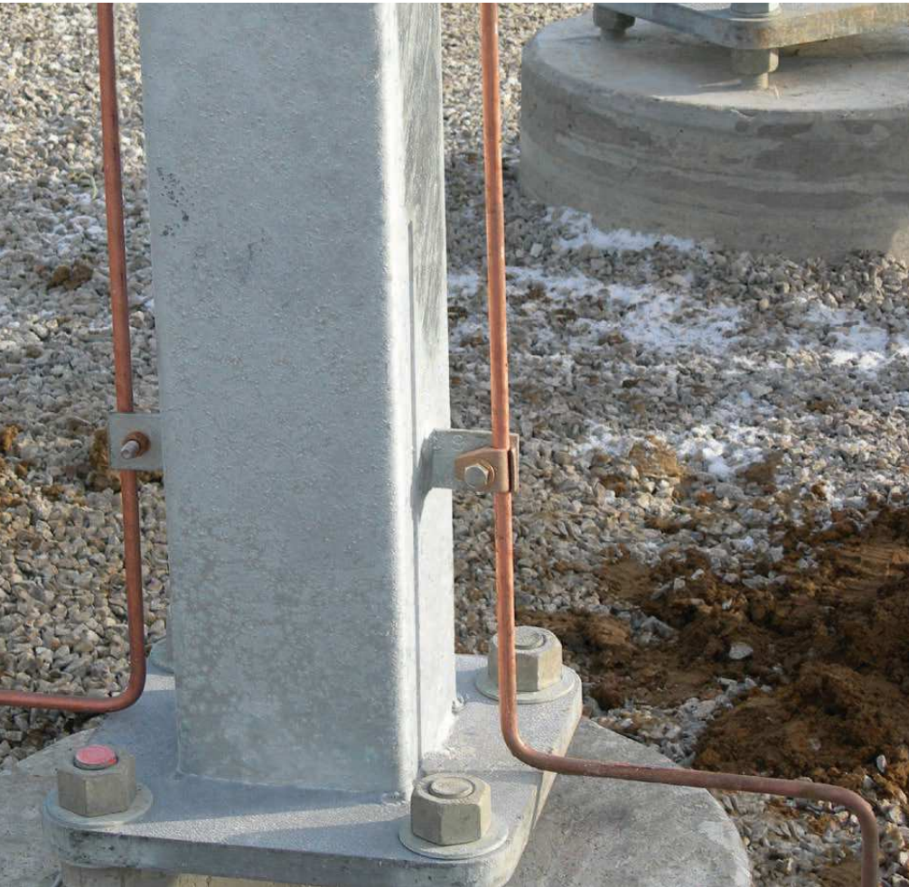
Substation earthing riser
