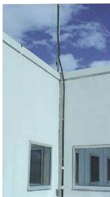
The Ericore Downconductor is easily retrofitted to existing structures. Inset: nVent ERICO Lightning Event Counter (LEC V) installed to register strikes to System 3000.
