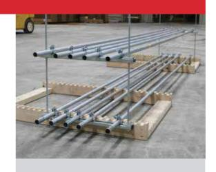
The spacing between pipes across the channel needs to be the same so that they meet up with each other when the individual runs are installed. It is recommended that installers use custom wooden jigs with notches at the spacing for each piece. They can be easily made on the jobsite with pieces of wood and customized for individual situations.
