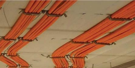
Material: Spring Steel Finish: nVent CADDY Armour
