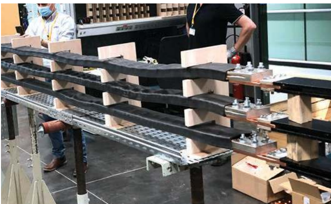
Temperature rise test sequence pictures and probe/temperature sensor all along the installation
