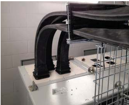
Example of individual cut out on nonmagnetic plate
