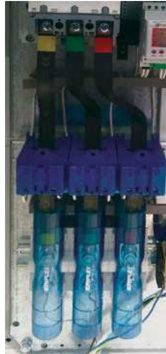
Application pictures: IBS & IBSB Advanced connected directly on ERIFLEX Power terminal and power blocks
