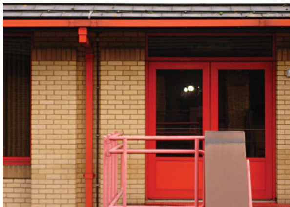
Figure 54. Example of poorly located a down-conductor.
