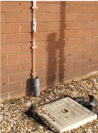
Figure 51. Typical down-conductor connectors.
