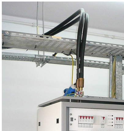
Figure 113. Incoming antenna circuits require protection.
