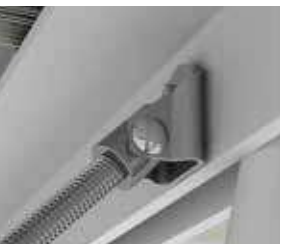
Branch Line Restraint Structure Attachment to Steel CSBBRS1MEG – p. 37
