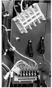
Close-up view of terminal block sub-assembly
