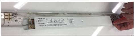
Step 1: Connect mains line "L" to fuse with one wire
