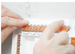
Snap the marking strips into the holder.
