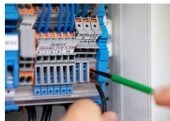
Conductor termination
